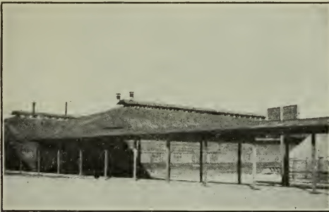
FIG. 12.—Hospital wards, Base Hospital No. 2, Fort Bliss, showing monitors along ridge and panels in wall.
